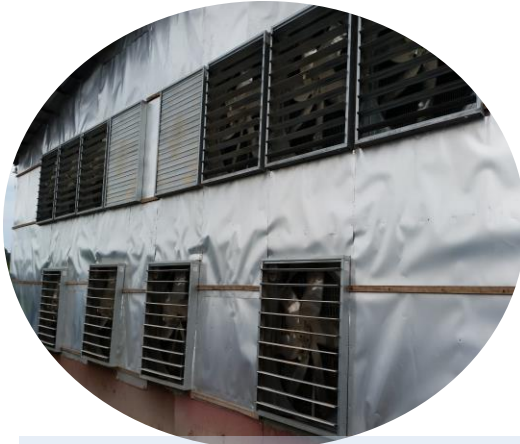
Efficient ventilation system
