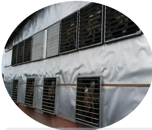
Efficient ventilation system
